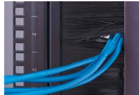
RU positions are numbered front and back, assisting with quick equipment installation
