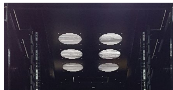
Cutouts for fans and large cable access in the roof
