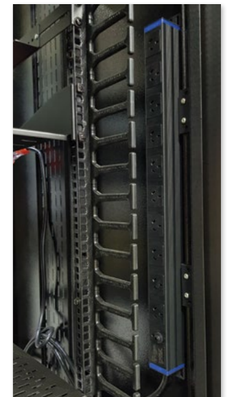
Vertical power rails can be mounted on uprights to save RU space
