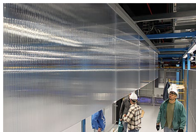
Installation of SPS
